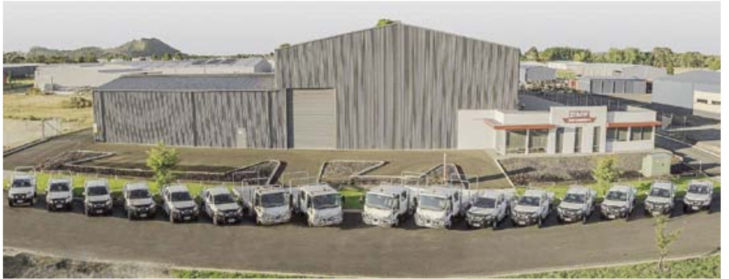
DMK Engineering's Mount Gambier base at Bodey Circuit.
