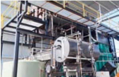
CARBON NEUTRAL: Roundwood Solutions on-site boiler converts waste wood into a multi-use carbon product.
