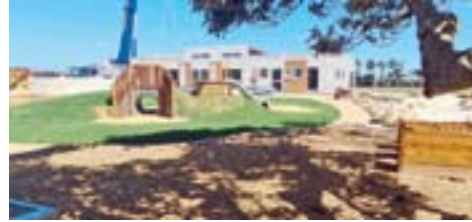
INSTANT PRESCHOOL: Six pre-fabricated modules were craned into place to form the new Moorak preschool this week.
