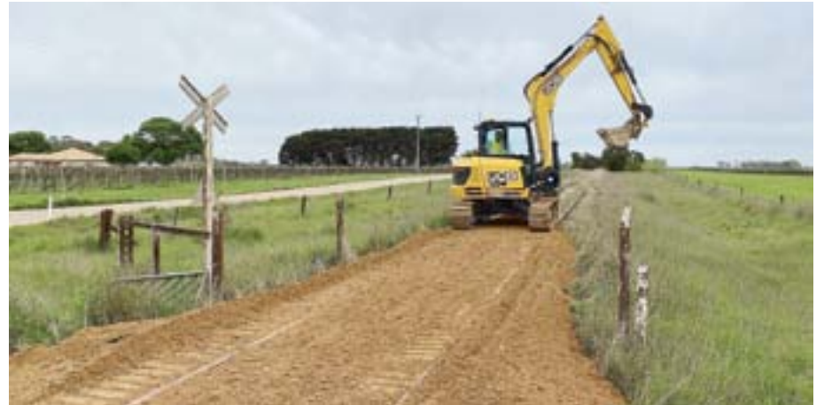
CONSTRUCTION CONTINUES: Work underway on Coonawarra Rail Trail.
