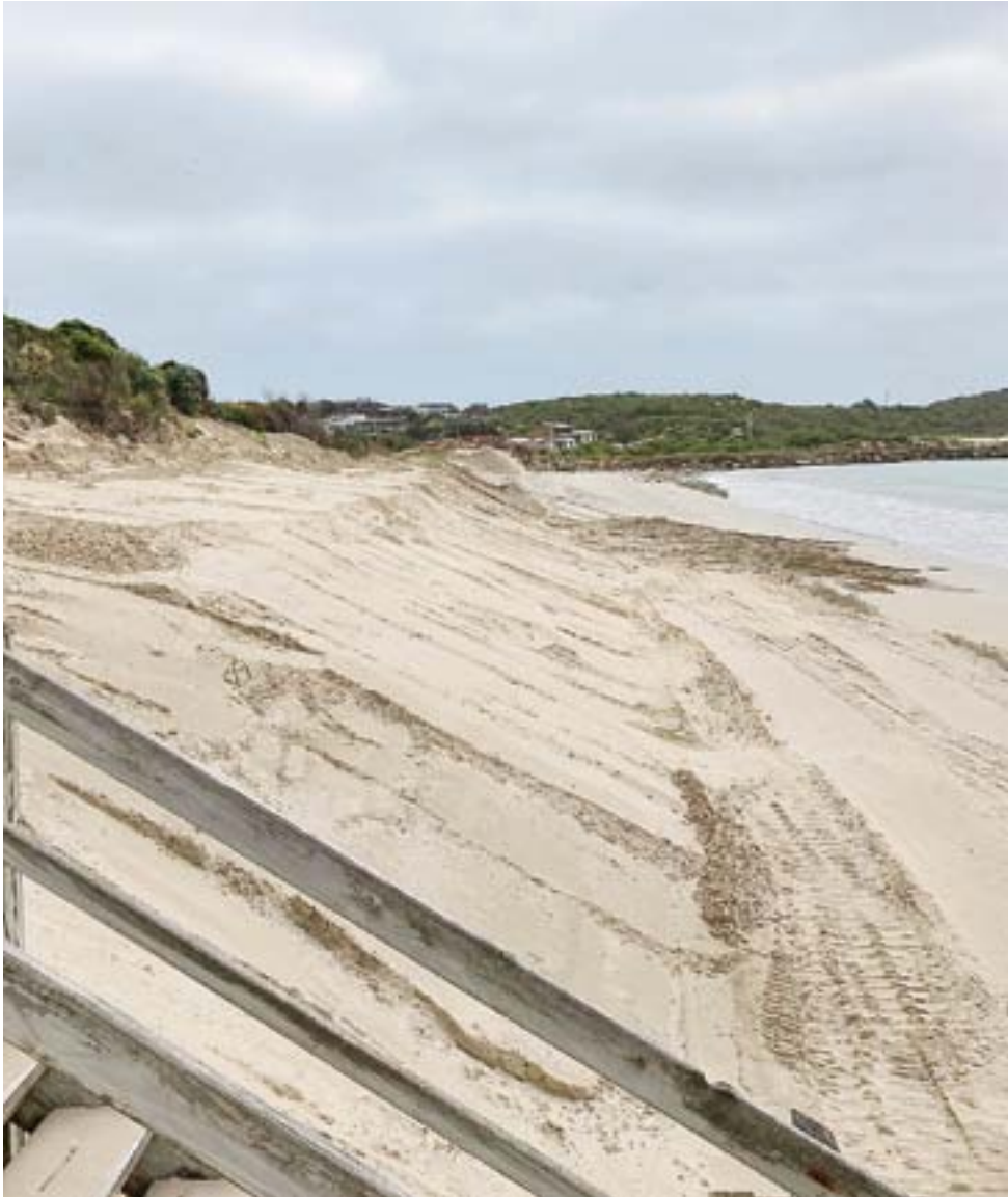
SAND ADDED TO SOUTHEND BEACH: The result of erosion remediation work completed recently. Pictures: WATTLE RANGE COUNCIL
